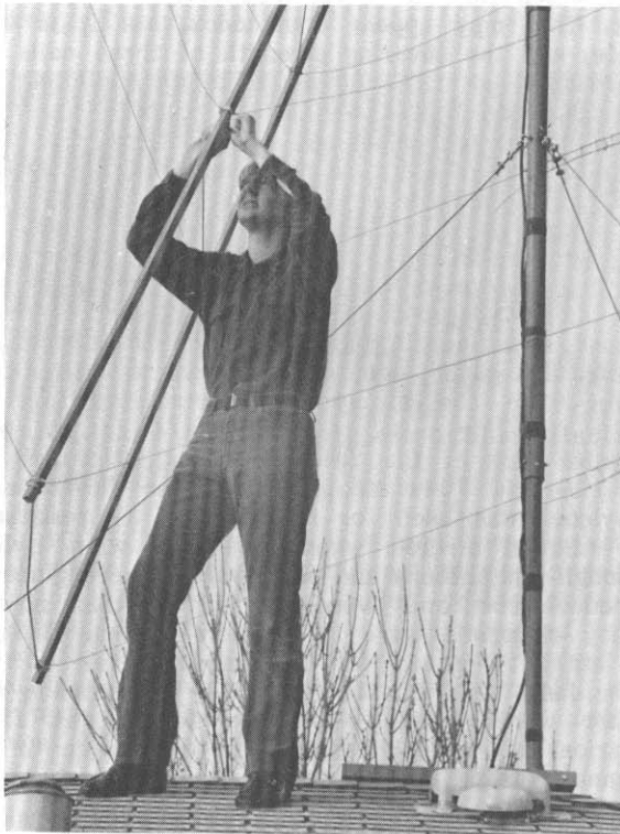
Fig. 5 -- NØART stands on the roof to add 12 polyester cross ties by rotating the quad in the vertical plane. Polyester is strong and stretches very little. It is also highly resistant to sunlight.
